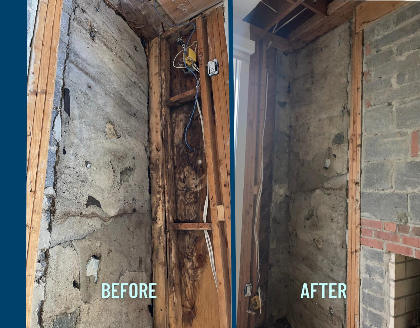
Here's the live work environment, there were 7 air scrubbers and 3 dehumidifiers set under negative pressure inside of a large containment to facilitate air quality improvements
